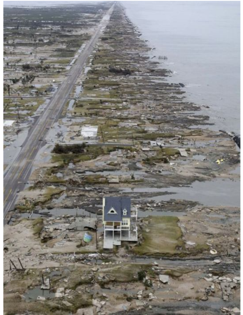
A picture of the coast near Gilchrist, Texas, after Hurricane Ike in 2008. This home's owners lost their previous home in Hurricane Rita in 2005. After Rita, they decided to build their new home to withstand a Category 5 hurricane. After Ike, it was the only coastal home left standing.
